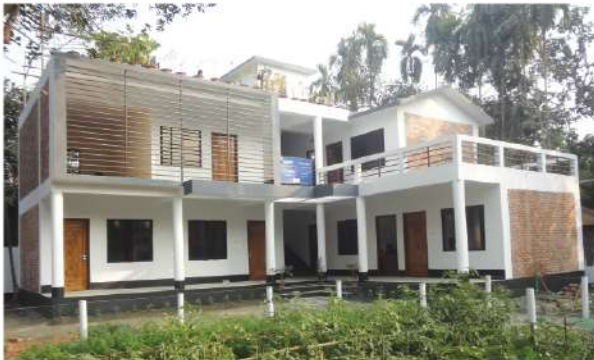
Sarishabari Project Office, Jamalpur
